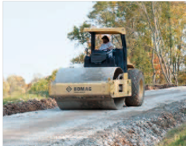
Effective and consistent compaction.
